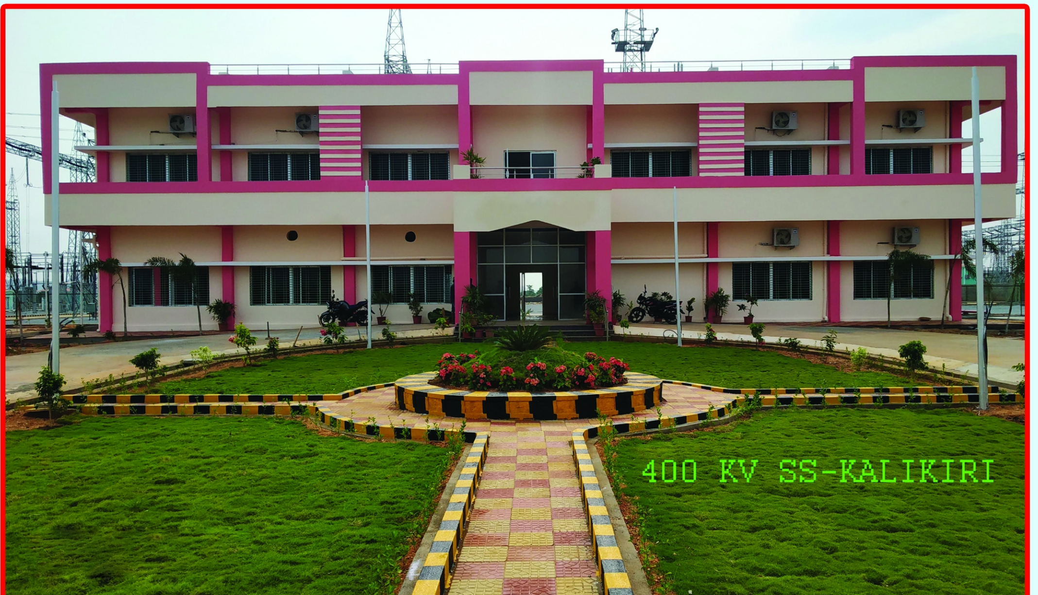
Kalikiri 400 KV Sub Station (Chitoor District)
