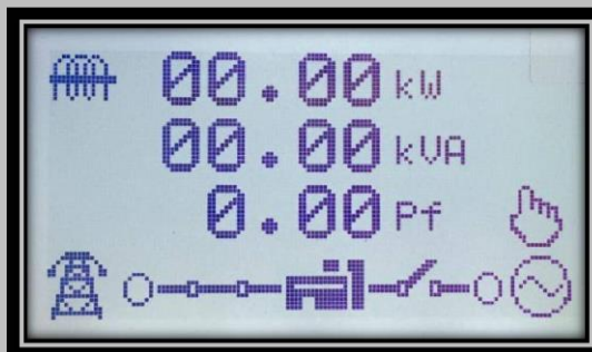
Combined Active Power, Apparent Power & Avg. Power Factor
