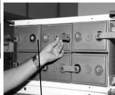
Remove Inter cell connectors
