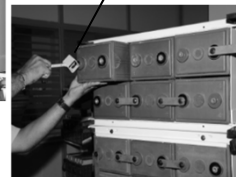
Remove the cell from tray by using cell puller
