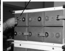
Release inside pressure by opening vent cap
